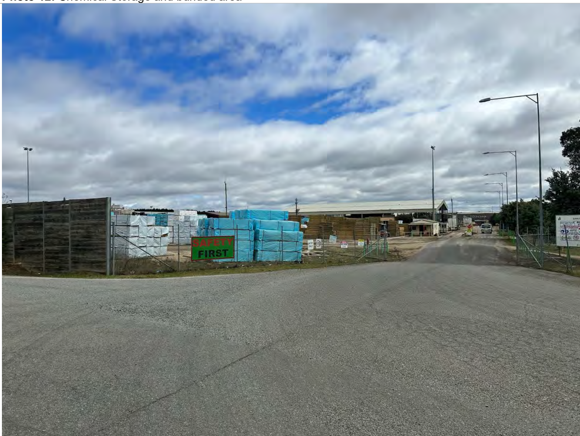
Photo 13: Site exit point with no mud tracking
