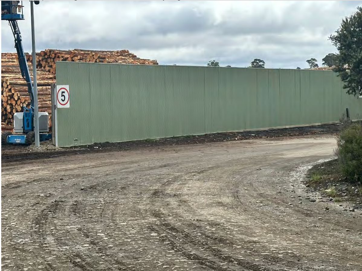
Photo 2: Acoustic hoarding and speed restriction signage
