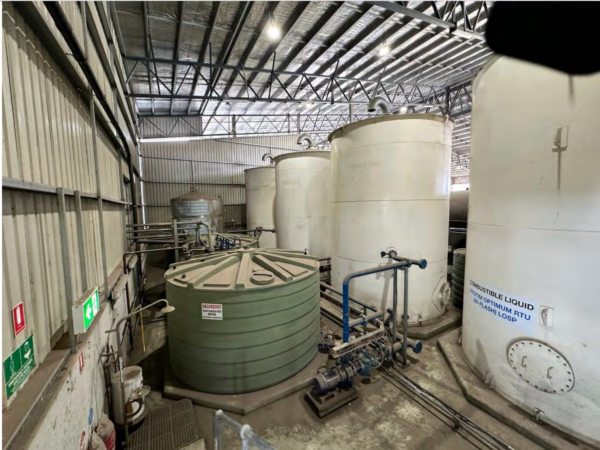
Photo 12: Chemical Storage and bunded area
