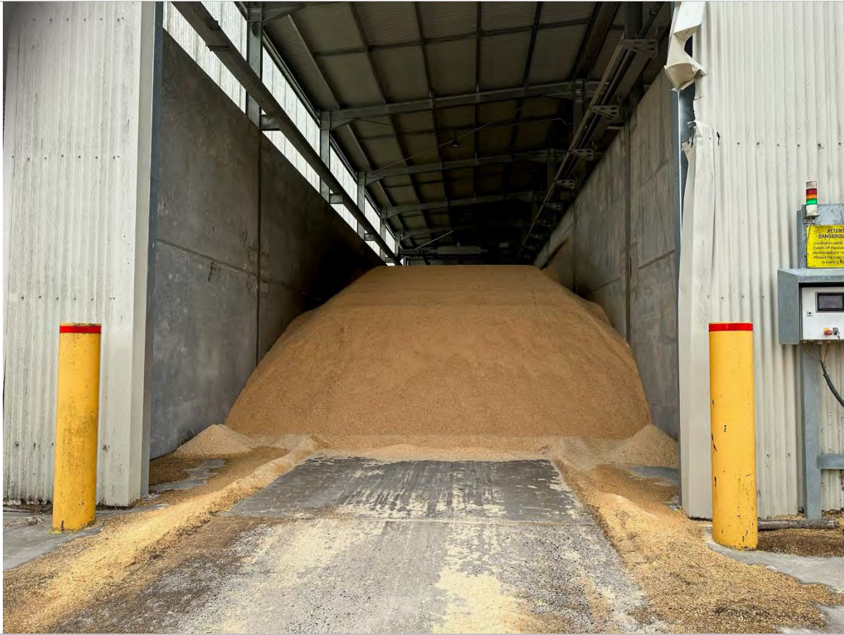
Photo 3: Sawdust stockpile stored for boiler fuel
