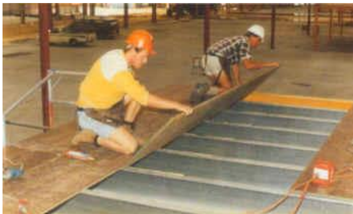
Sheets should be pushed firmly together by hand - mechanical cramping is unnecessary
