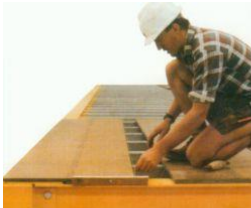
A string line should be set to ensure the first sheet is square with the joist.
