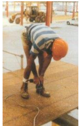
Particleboard flooring can be quickly fixed to timber or steel joists with nails or screws using hand or power tools.
