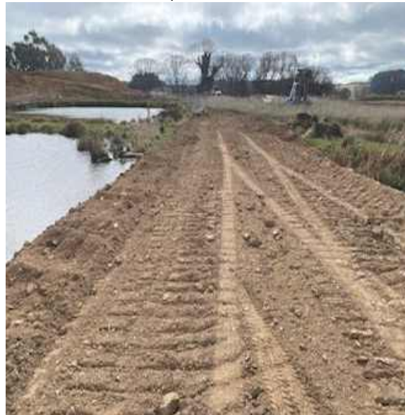
Earthworks to 'close' ponds
