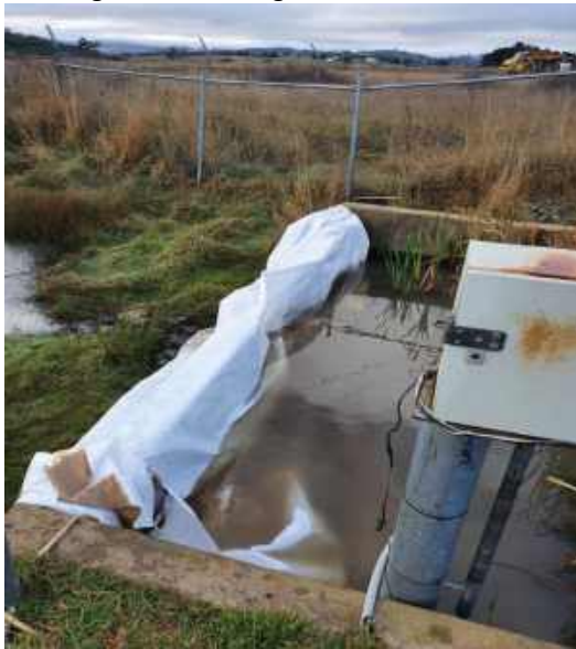
Blocking V-notch with geofabric
