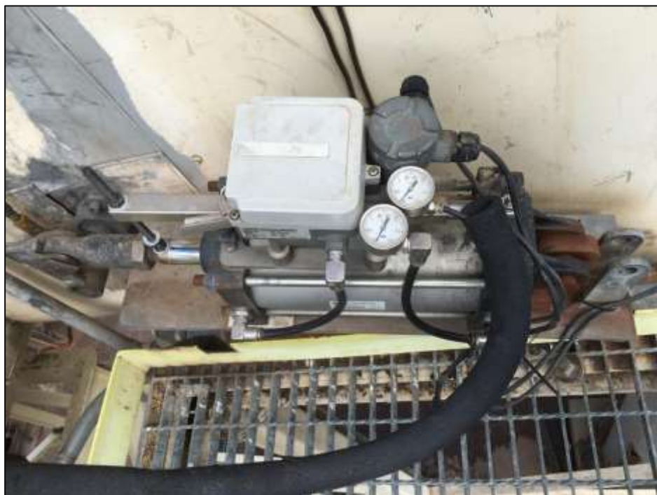
FIGURE E-4 CONTI-2 HEAT PLANT OUTLET BYPASS DAMPER CONTROLS (DAMPER SHUT)
