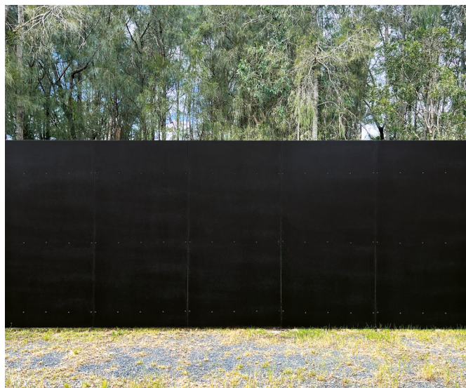
12mm – Temporary hoarding panelling
