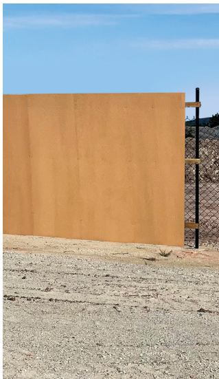
12mm – Temporary hoarding panelling
